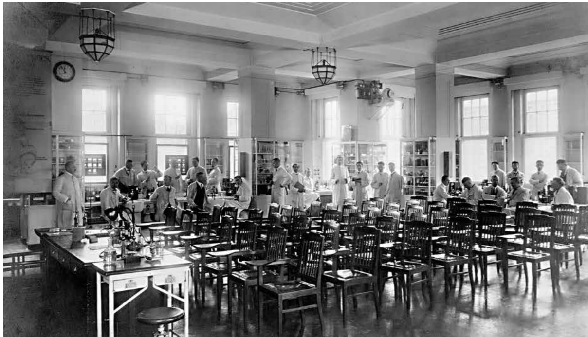
Historical photograph of the course hall
